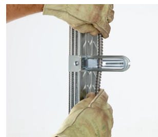
Insert cables to be secured
