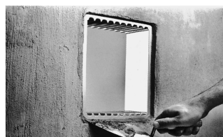
1. Cast, grout or weld the one-piece mounting frame into masonry or steel surface.
