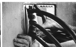
2. Feed cables/conduit through the frame.
