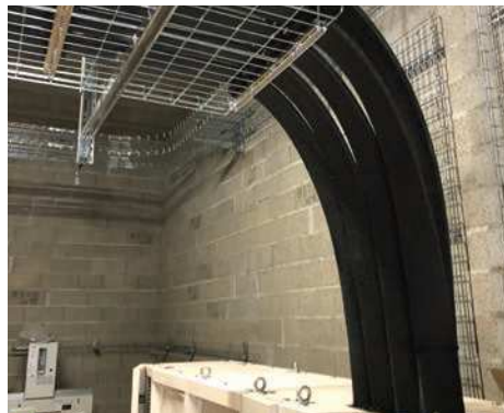
Rendering of Flexbus installed under the raised floor of a clean room
