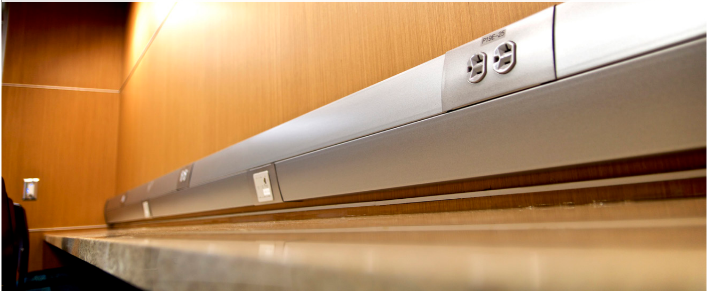
SURFACE RACEWAY
