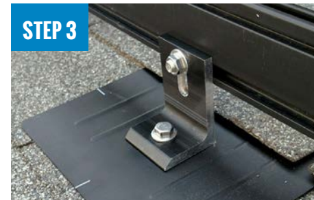
ATTACH L-FOOT TO RAIL
